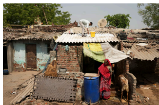
A man applies reflective paint to the roof of a shanty home in Ahmedabad, India, to reduce indoor heat. Photo: AP
